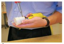
**3** Insert bare wires into their corresponding color-coded terminals. Make certain there is not wire insulation under any terminal clamp. Tighten the screw clamps to 14-20 inch-pounds torque.
