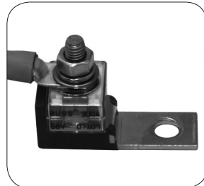
Fig. 3.9. MRBF Fuse and Positive cable fixed to the CFBAR
